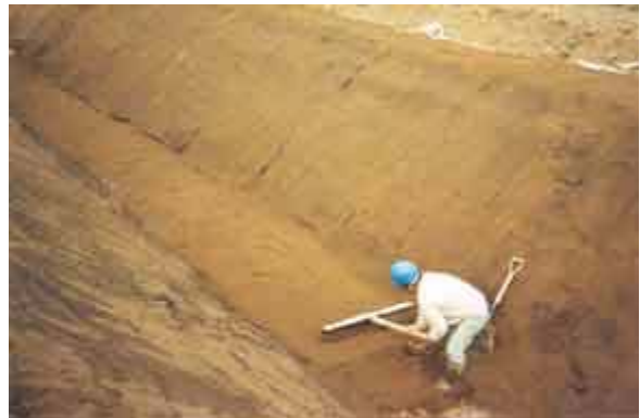
Filling of the geomat with organic soil
