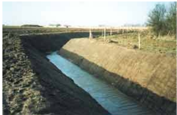
Completed channel section during the germination process
