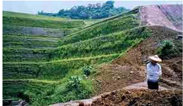
Reinforced slope two months after construction
