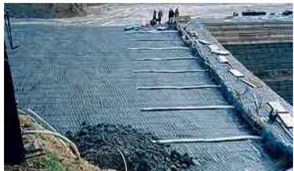
Reinforced slope two months after construction
